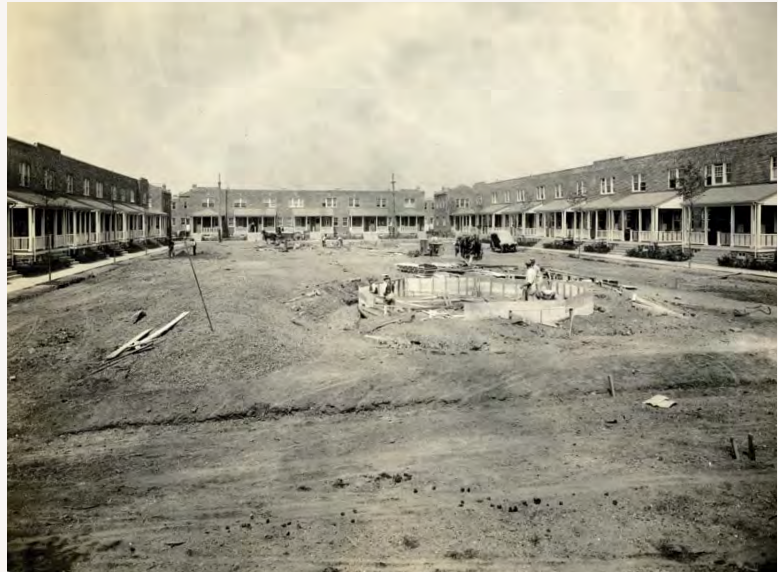
Looking west at the 700 block of Mollbore Terrace under construction, May 1919.
