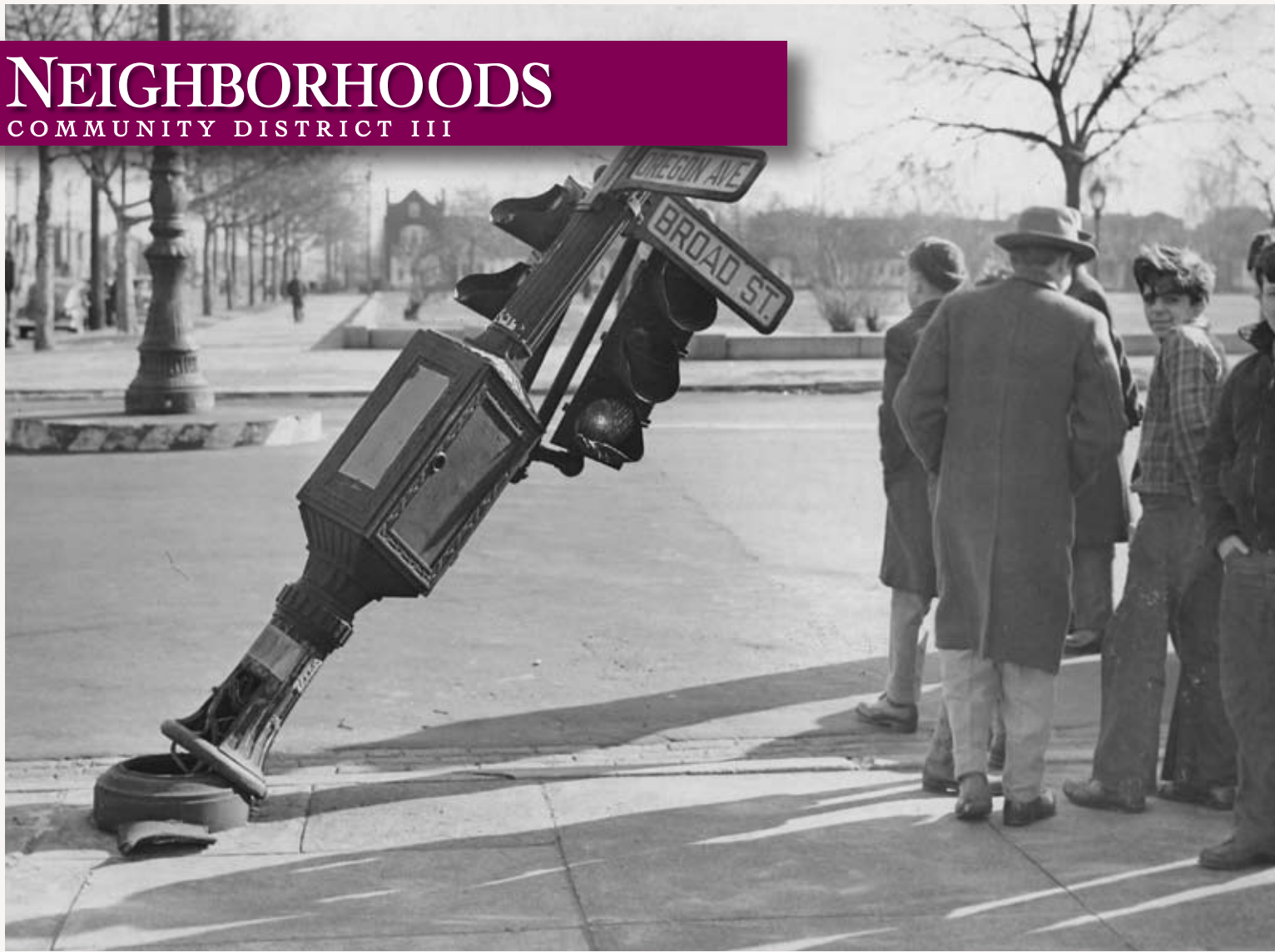
A damaged traffic signal at the intersection of S. Broad Street and Oregon Avenue, December 11, 1944.
