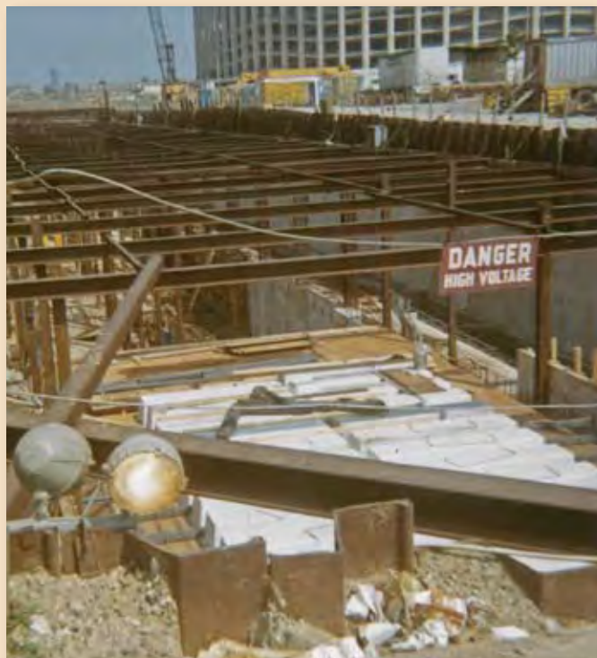
Subway construction next to Veterans Stadium.
