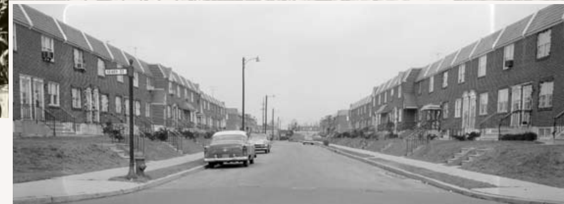
View of S. Juniper Street, looking north from Geary Street, December 31, 1956.
