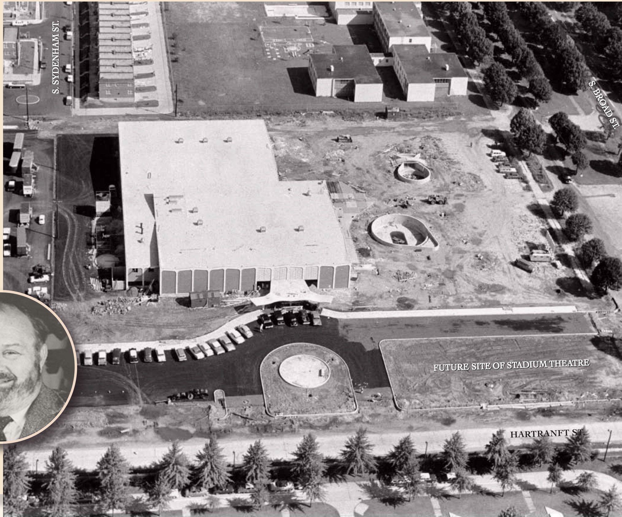
Aquarama under construction, July 30, 1962.
