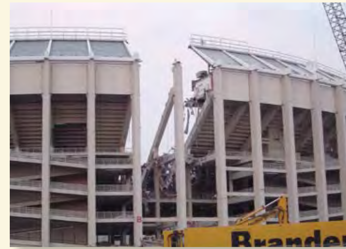
Contractors prepare the Vet for implosion, March 9, 2004.
