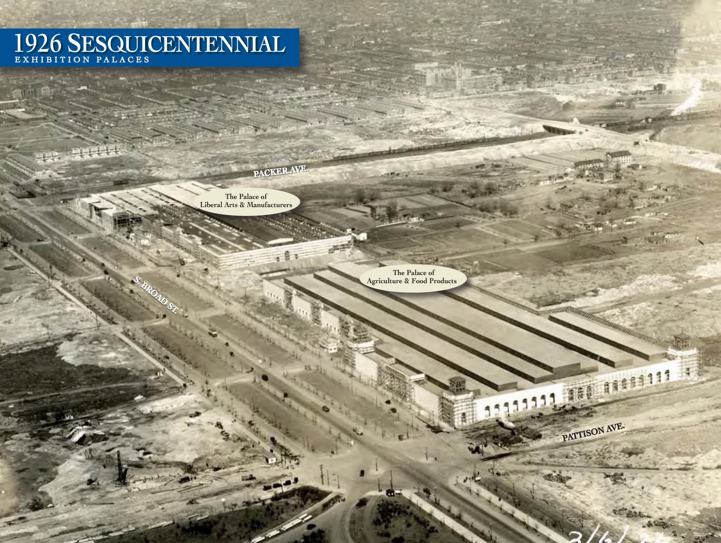
Construction of the Palaces, March 6, 1926. The Palace of Liberal Arts & Manufacturers was located on the southeast corner of S. Broad Street and Packer Avenue, today's Community District 1. The Palace of Agriculture & Food Products was located on the northeast corner of S. Broad Street and Pattison Avenue. This is the current location of the Pattison Subway Station and Sports Complex surface parking lots. Homes in Community District 3 are visible at the top of this photo.
