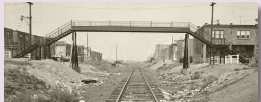
Views of the S. 17th Street pedestrian footbridge spanning the railroad tracks in 1952. Tunnels would later replace the footbridges to retain pedestrian access under the Schuylkill Expressway.
