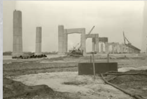
Looking west at the construction of the bridge approach piers, September 1955.
