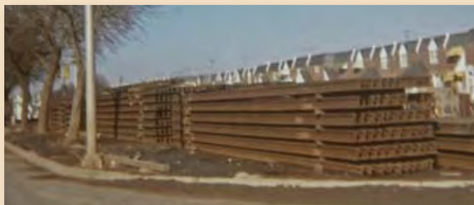
Subway construction supplies staged in front of District 1 homes.
