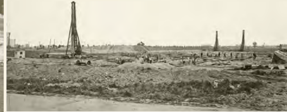
Construction of Municipal Stadium, May 18, 1925.
