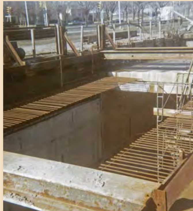
Subway construction at Broad and Geary Streets.
