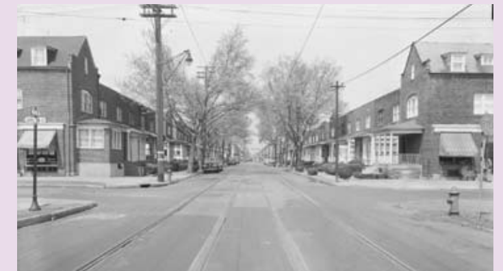
Looking north on S. 7th Street at the intersection of Johnston Street, April 22, 1952.
