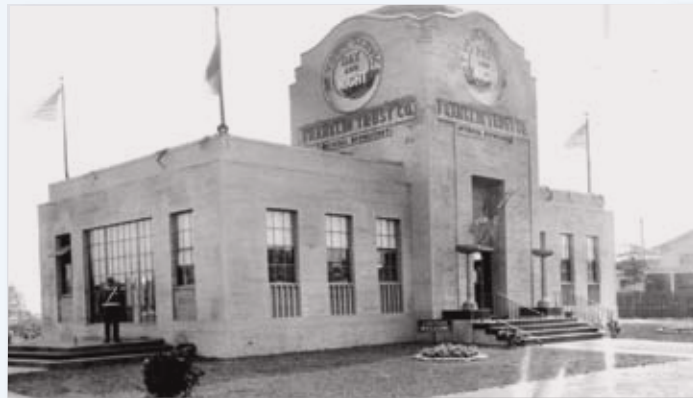
The Franklin Trust Company building was located in the Nuremberg section, took only 24 days to construct, and served as the official bank depository for the Exposition. The company's trademark logo "At Your Service Day and Night" advertised the bank's ability to serve the public until midnight daily, even on holidays.
