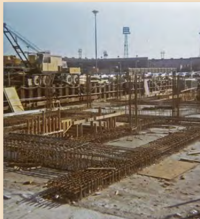
Subway construction with JFK Stadium in background.
